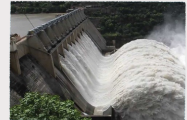
Nagarjuna Sagar Dam
