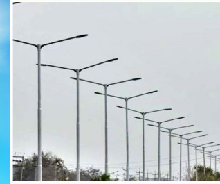
Electrification on main road
