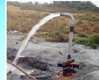
Bore water facility in common area
